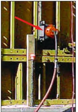
Special vibrator bracket was designed to clamp on to form stiffener.
